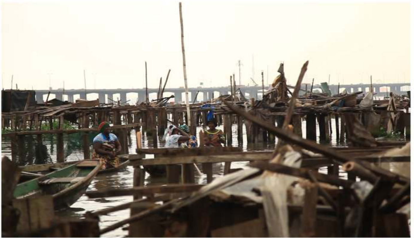
Destruction of Makoko 2012, photo Deji Arosho
